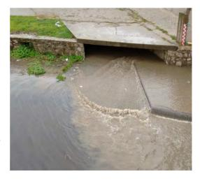
combined sewer overflows (CSO), which have a function to overflow the excess water during wet weather conditions (storm events) in order to protect the WWTP from overloading.
